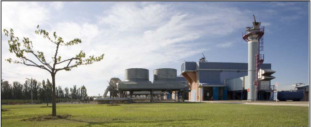
Station de compression de GRTgaz
